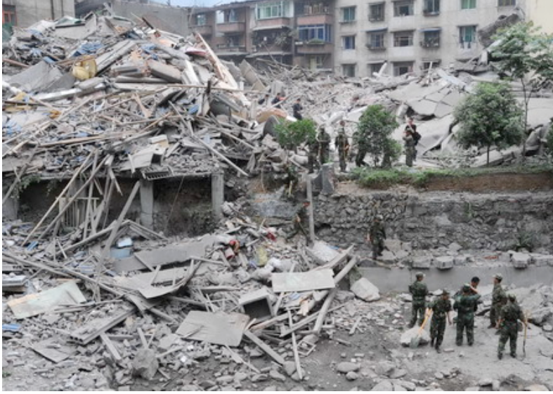
Figure 6 : Damaged buildings after Si Chuan earthquake. People's Daily, May 13
